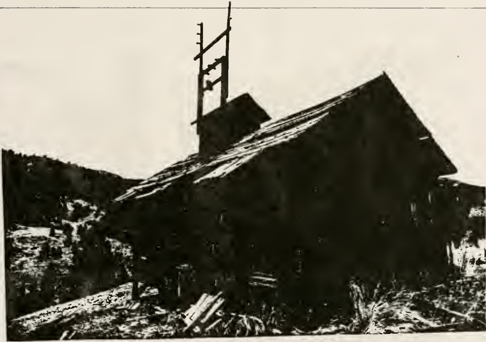
Figure 143. Electric substation (structure #54), northwest view.
